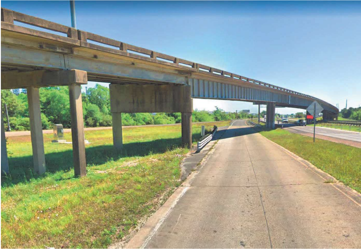
Figure 1 – US 90 Bridge over I-10
